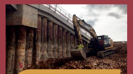
"Actions taken eliminated significant potential costs and resulted in more than 200 contiguous piles being completely defect free, with 100% vertical tolerance compliance."
